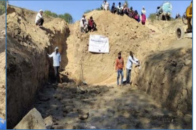
Check dams being constructed in Alwar district to catch and channelize rain water. Another sustainable initiative is to channelize and save water through a project of "Water conservation through installation of rainwater harvesting structures in the form of check dams and gabion structures" in Alwar, Rajasthan. PFS has funded four check dams and two gabion structures to improve ground water situation in the area.
